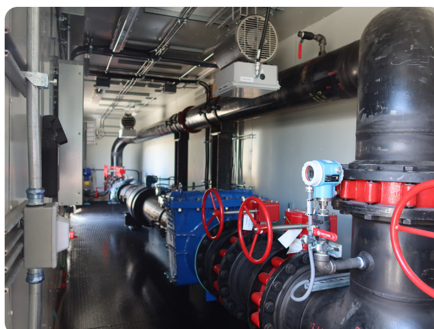
Pressure control container for a mine site. Several pressure control and flow control containers were delivered for this project.
