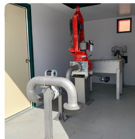
Septage receiving container for a wastewater treatment plant. Designed for extreme cold weather operation.
